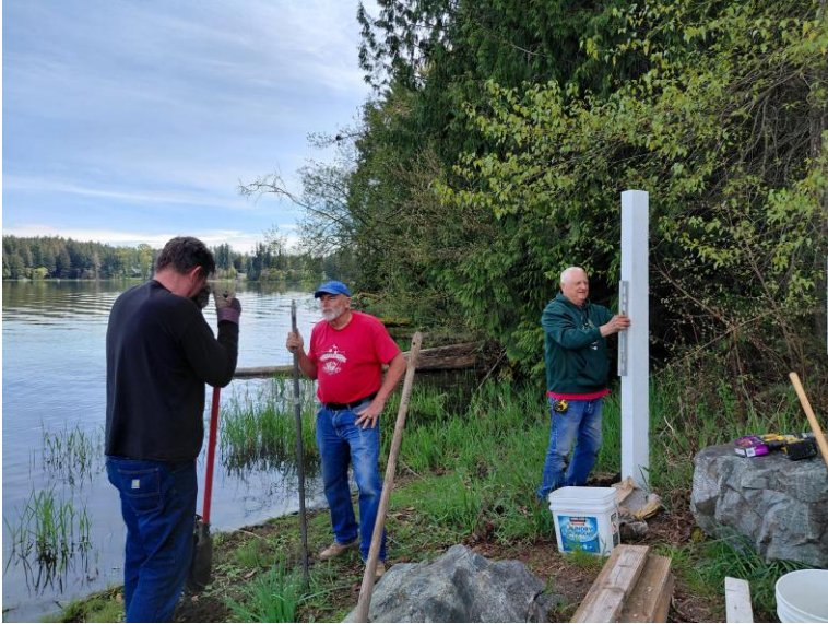
On 18 April 2026 Barry, Frank, Jim, & Carl installed the signposts for the Boat Launch Safety Sign at the DFW Boat Launch.
