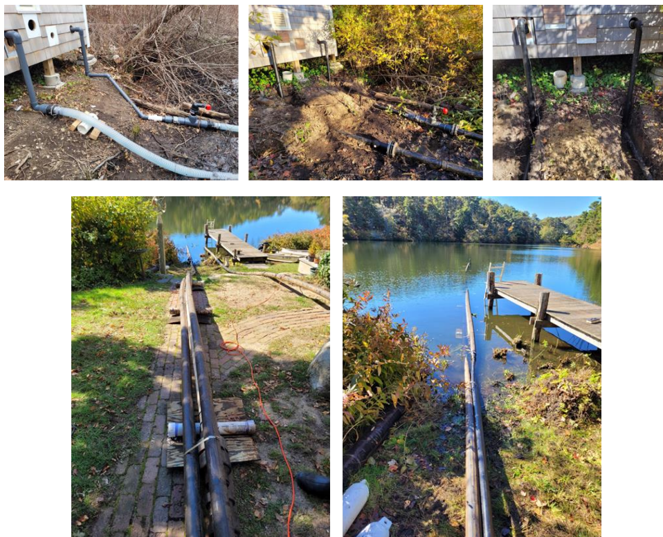
Figure 10. Updated piping on shore (top) and in the lake (bottom)
